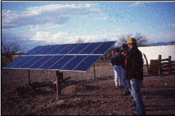
Figure 3. PV pump at Rancho Jeromin in Chihuahua.
