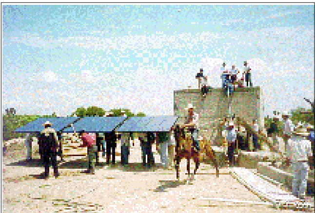
Figure 9. El Reventon PV pumper in San Luis Potosí
