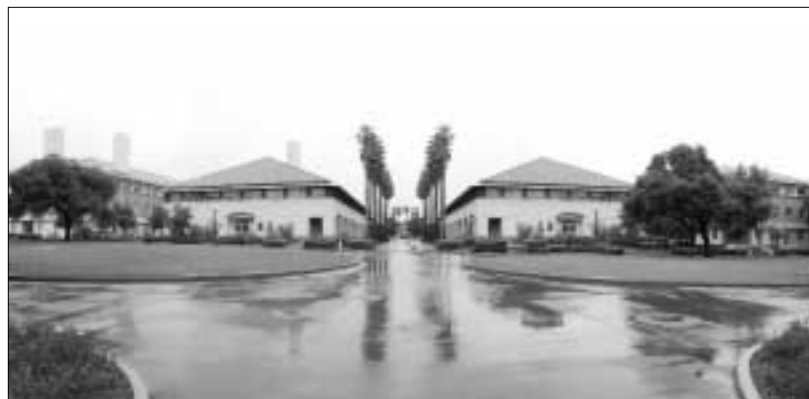
Varian 2 – to be completed by the end of 2005
