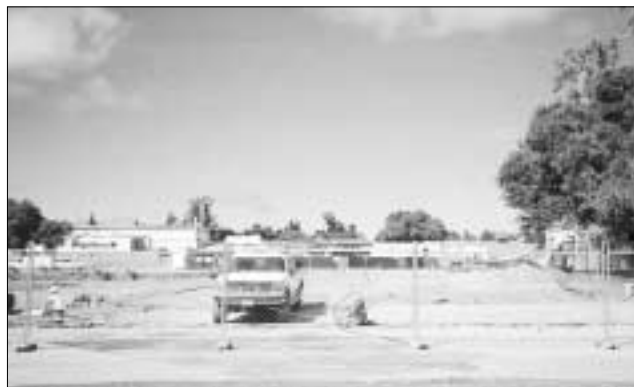
Photos of Tank deconstruction.
