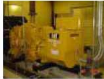
Turn on emergency generator (can use as monthly generator test)
